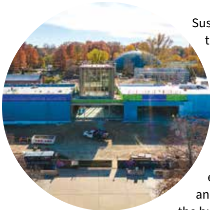
Construction progress, winter 2021
