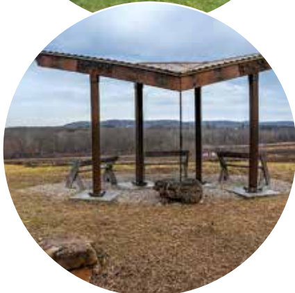
(top) American Wild Ensemble performs at Bascom House (bottom) McMillan Prairie Overlook construction
